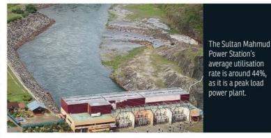
The earth core rockfill type Kenyir Dam is elevated at 155m above sea level, with a maximum flood level of 153m. Its maximum operating level is 145m while its minimum operating level is 120m. If the dam's water level exceeds 145m, the excess water will flow out through the ungated spillway, which has a maximum capacity of 7,000 cubic metre per second. The Kenyir Lake reservoir has a surface area of 369 sq km, with
